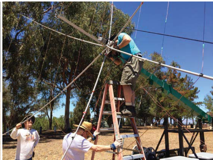
Attaching the K4KIO Hex Beam to the tower trailer.
