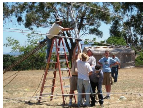
Ready to lift the SSB Tower
