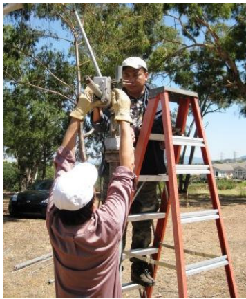
Setting up the Satellite Antenna
