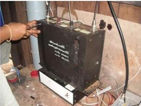
Here we see the home made repeater controller. It consists of an ICOM IC2800H and a MOTOROLA radio. The controller is very simple, nothing fancy at all – no features like we have here. No need to have CW ID or tone or anything. By regulation, Amateur radio is still not allowed to have a PL Tone or TSQ to be installed on any Transceivers.
